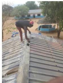
Fixing loose panels
