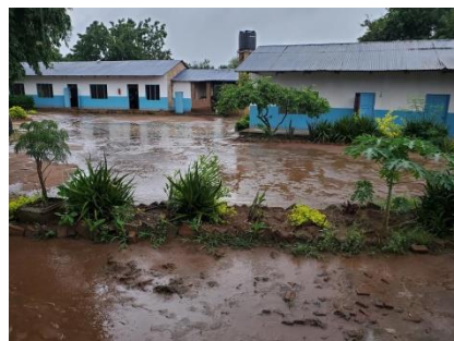
Flooding around the college buildings
